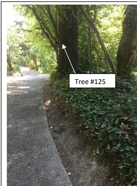
Photo 3. This is the neighboring Driveway to the south and graded cut slope potentially impacting roots.
